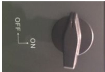
Figure 109 - Photovoltaic disconnecting switch
