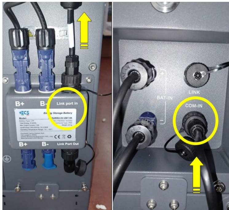
Figure 132 - Communication connections: BDU and first battery module
