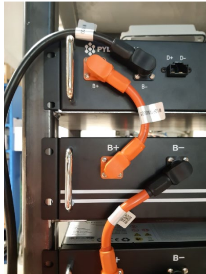
Figure 44 - Power connection (positive) between the BMS and first battery module
